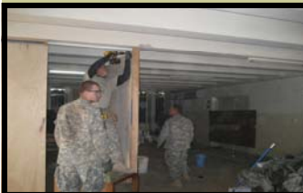
A Co Soldiers making improvements to the JSS in Tarmiyah
